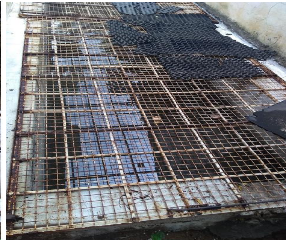
Rain Water Harvesting Pits In GRIET Campus
