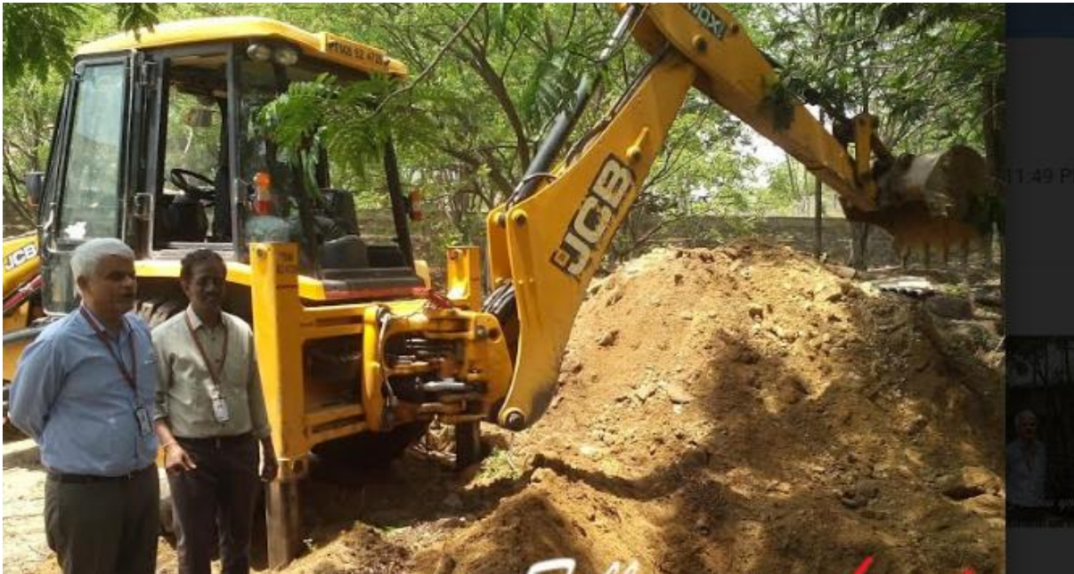
Rain Water Pits Execution : Monitoring By Director GRIET
