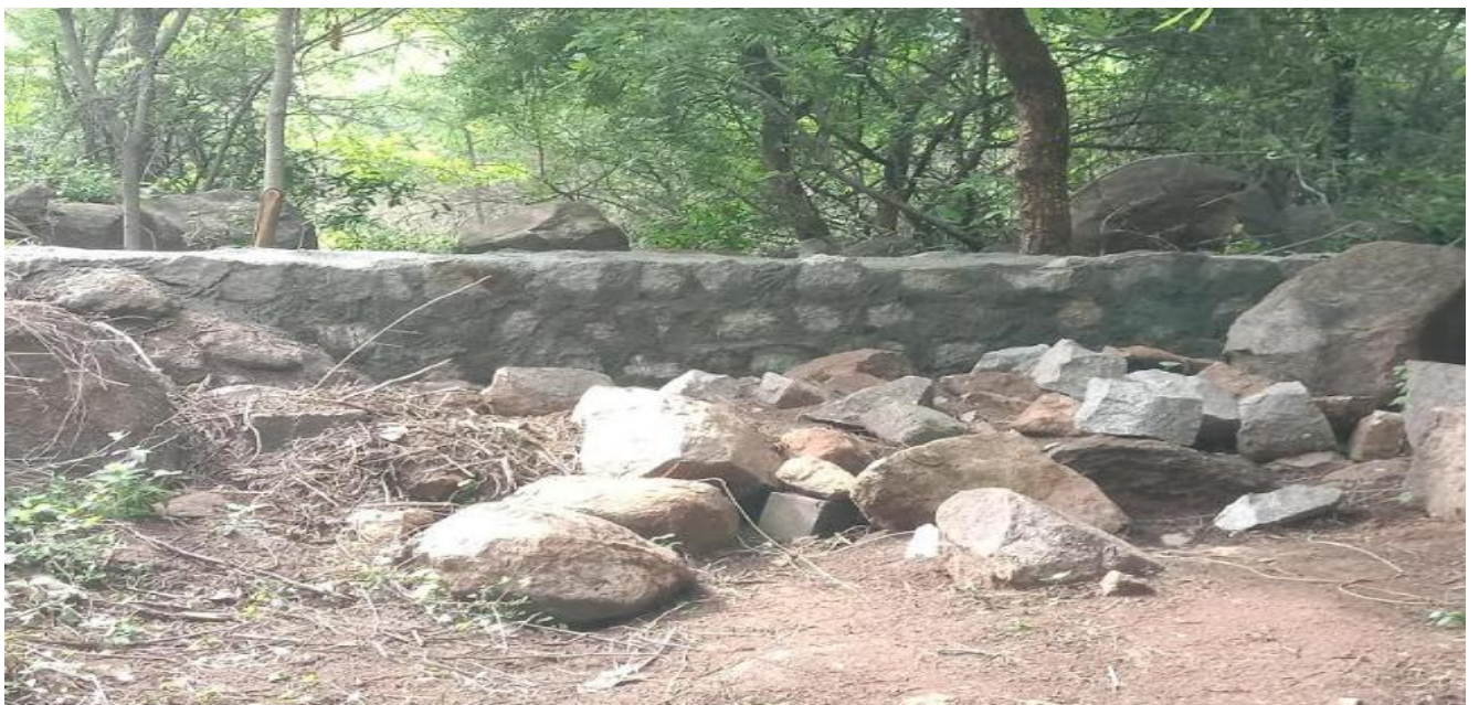
Construction of check dams Masonry
