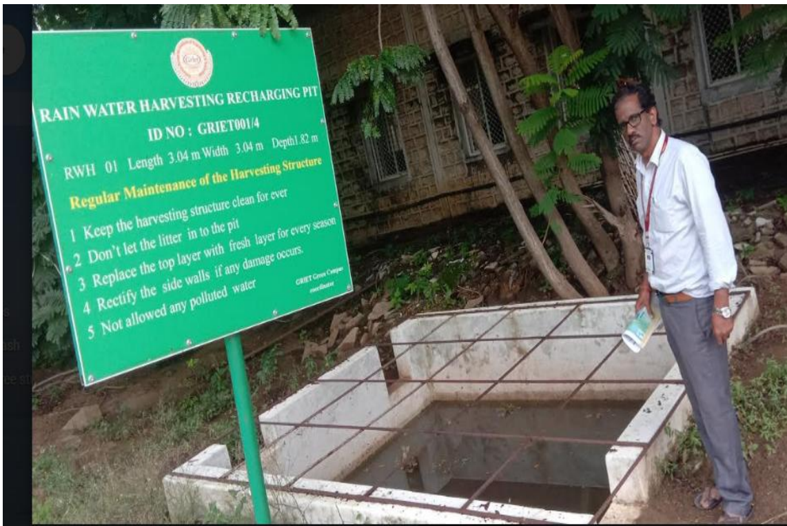
Rain Water Execution Monitoring By GRIET Green Campus Coordinator
