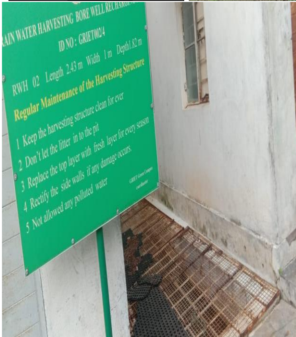
Bore Well Recharge Pits
