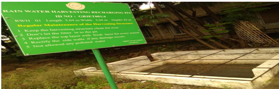
Rain Water Harvesting Pits In GRIET Campus
