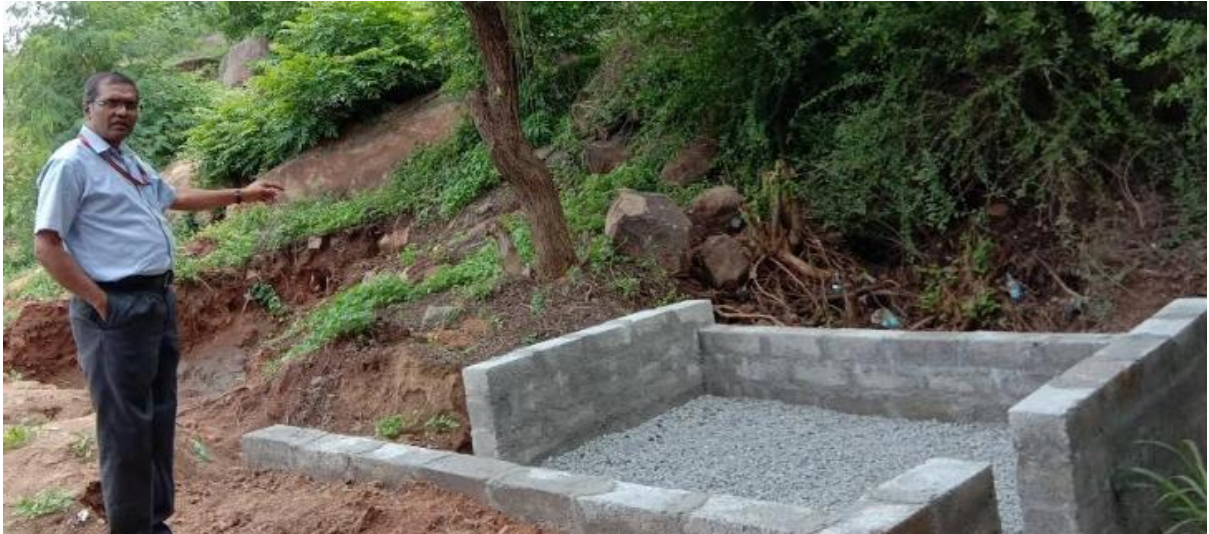
Rain Water Pits Execution is Monitoring By HOD Civil GRIET
