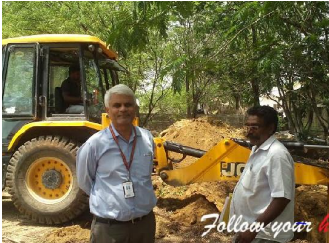
Rain Water Pits Execution : Monitoring By Director GRIET
